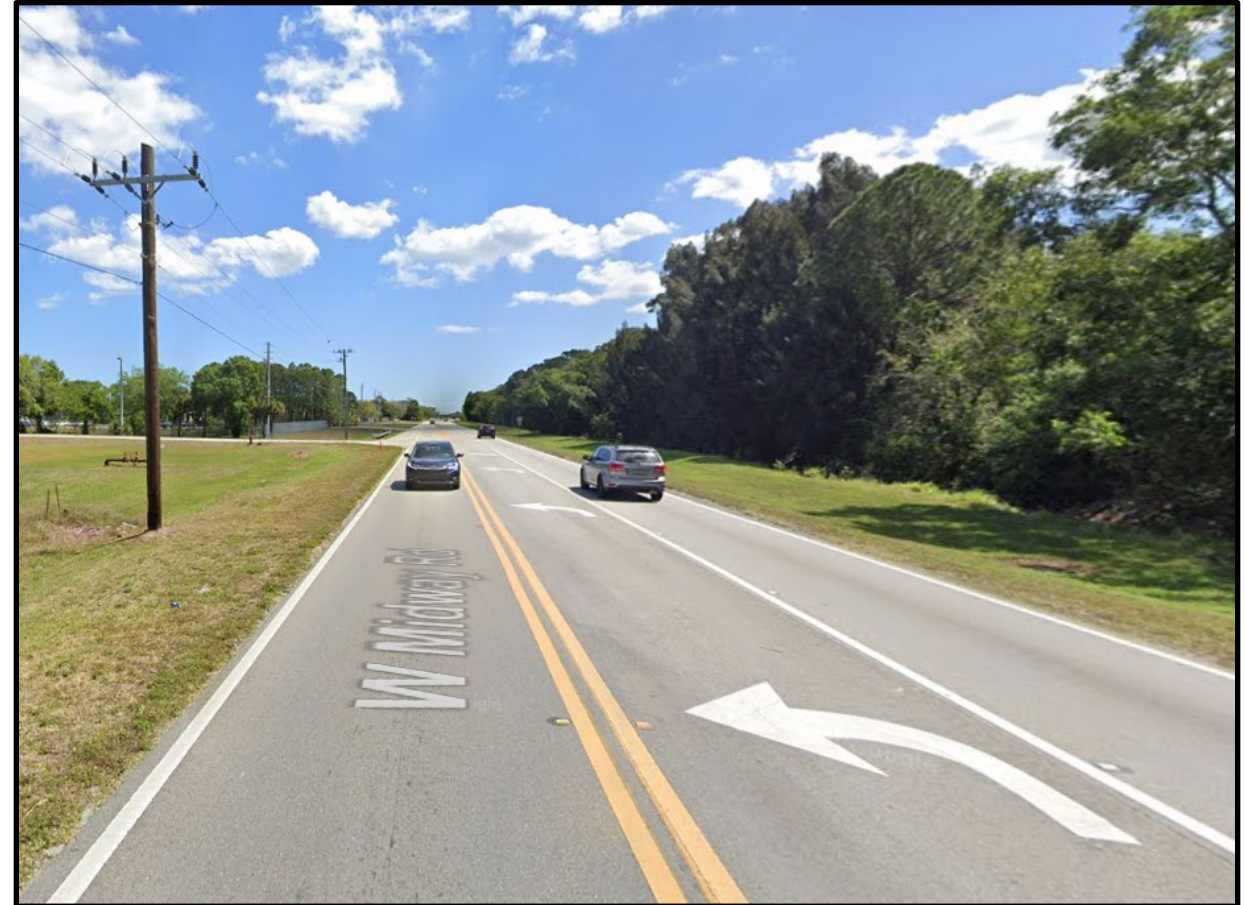
CR 712/Midway Road at Selvitz Road in front of the United States Post Office looking east (pre-construction)
