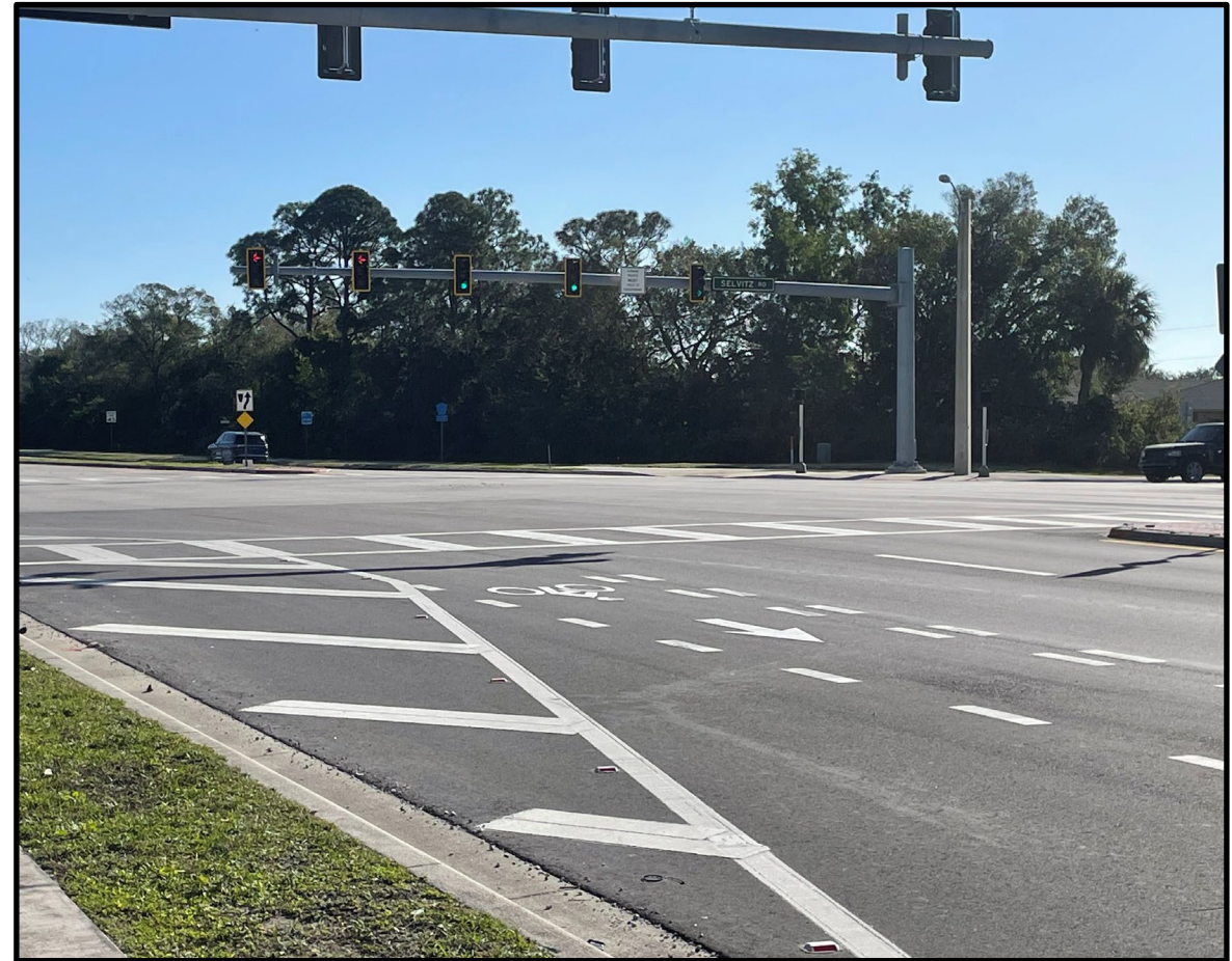
Intersection of CR 712/Midway Road and Selvitz Road looking west (pre-construction)
