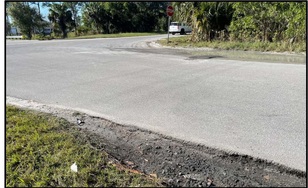
Intersection of CR 712/Midway Road and Jenkins Road (pre-construction)
