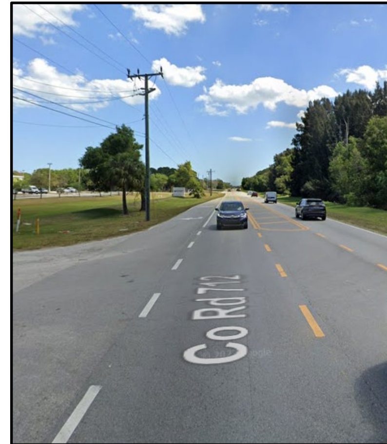
CR 712/Midway Road at Post Office Road looking east (pre-construction)
